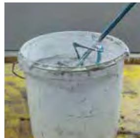
Do not stir hardened mortar a second time, but dispose of it instead.
